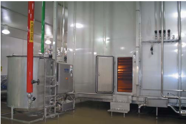
Recirculating Clean-In-Place (CIP) system
